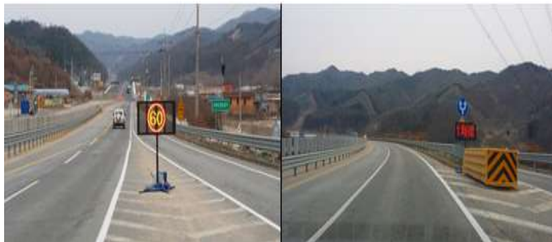
Figure 3 Variable message sign set up at 200m and 500m upstream of constriction section
