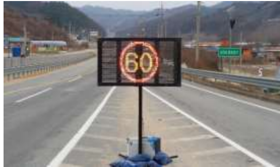
Figure 1 Variable message sign
